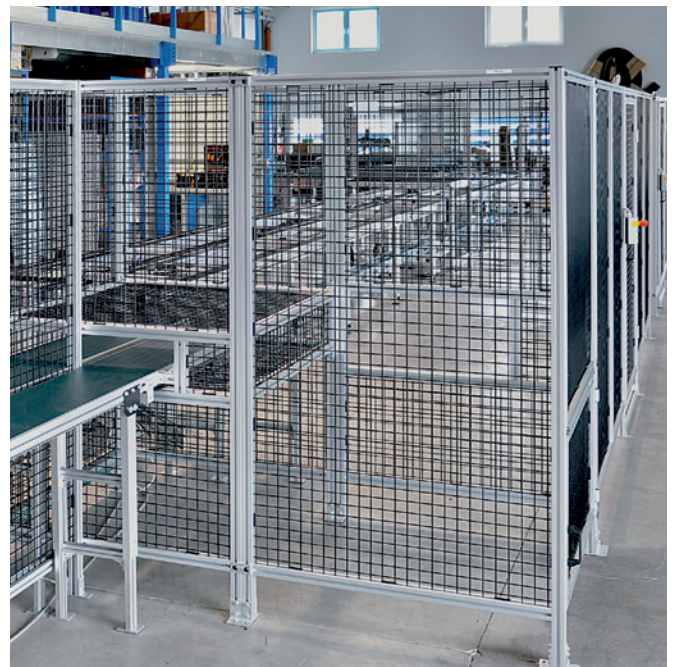
Perimeter guarding can be made standard or custom. Here the perimeter guard also includes a reach-in protection around the conveyor.
