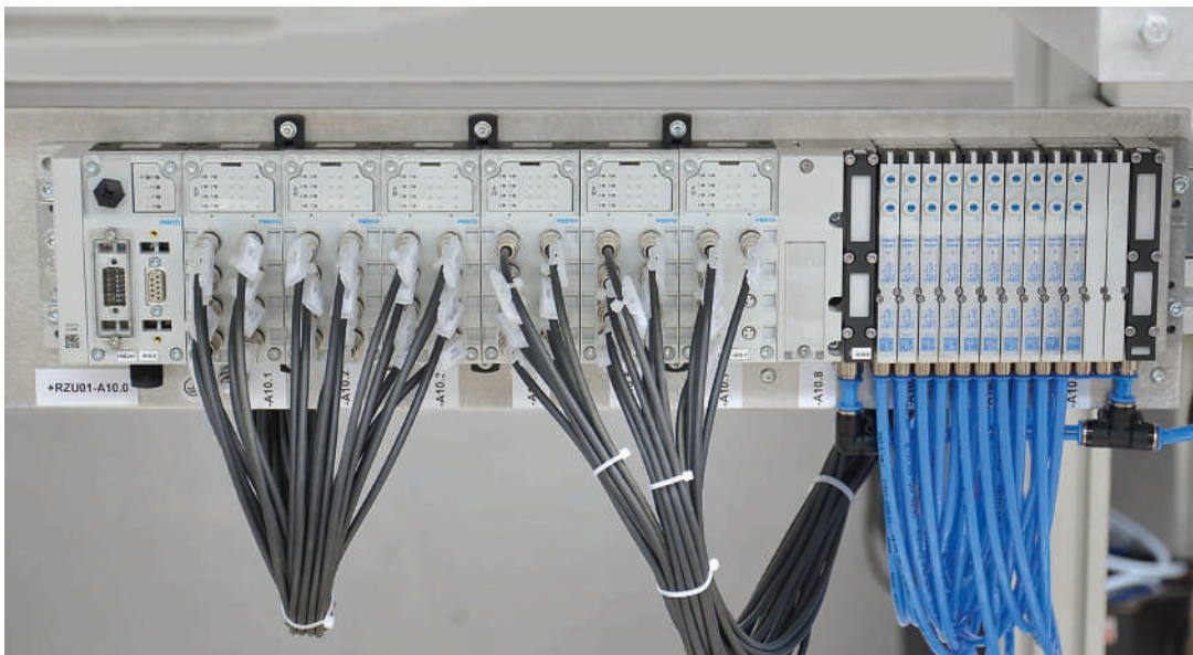
Valve terminal with input and output module
